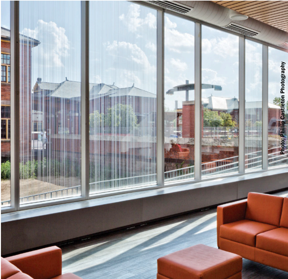
Humber College Centre for Entrepreneurship in Toronto incorporates AviProTek® bird-friendly glass by Walker Textures® glass, acid-etched on tinted Solarban® 70XL glass.
